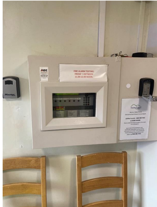
Addressable panel installed which is connected to an alarm receiving centre.
