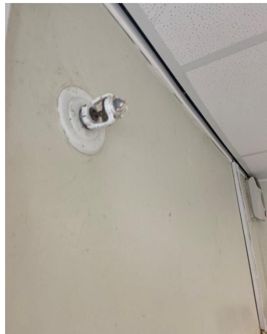
Sprinkler system is installed within communal area and self-contained flats. This is unusual in accordance with the British Standard.
