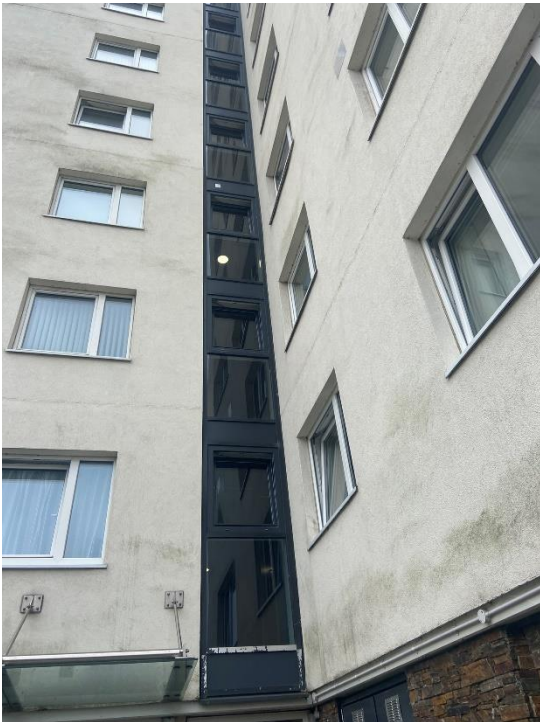
Spandrel panels run vertically the entire height of building in an isolated location.
