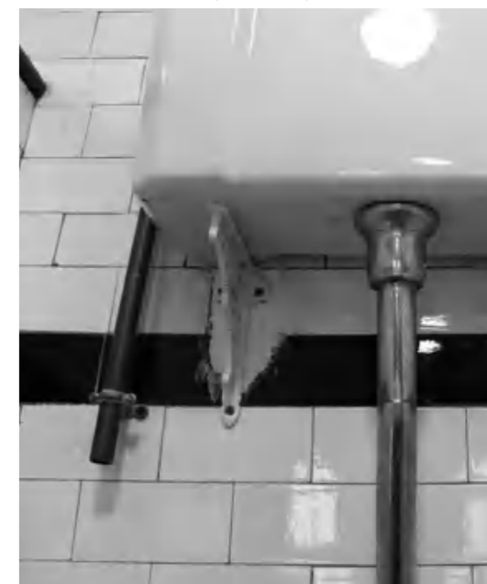
Typical Cistern Fixing / Damage
