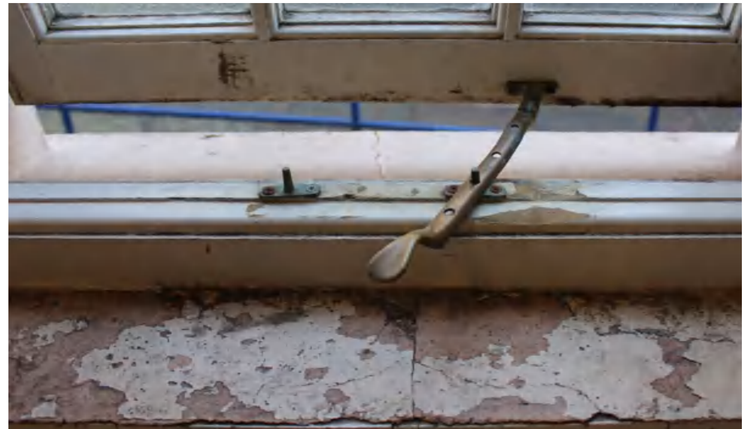
Window 07 - Typical Brass Stay and Localised Scarf Repairs to Stool
