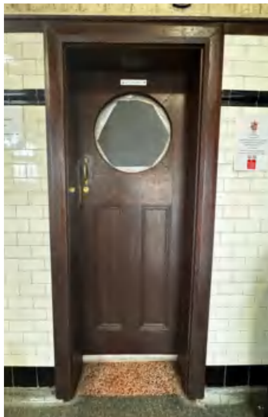
Door 13 Damaged Glazing
