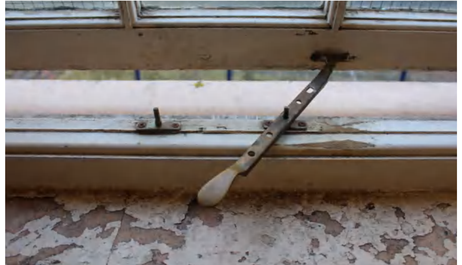
Window 07 - Typical Brass Stay and Localised Scarf Repairs to Stool
