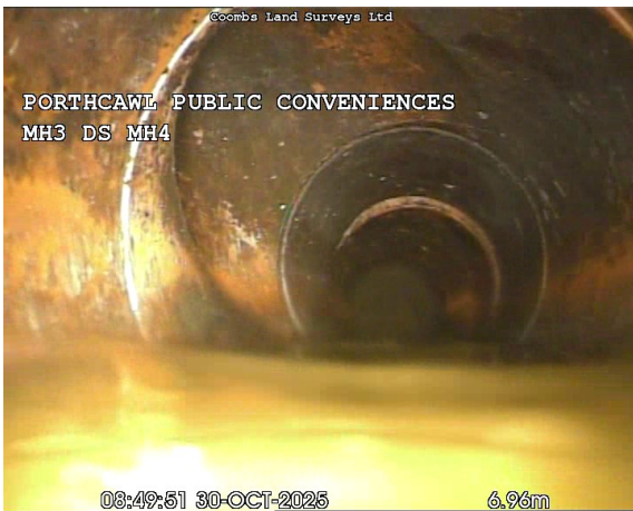
MH3X_32429f62-5b9a-4f69-b728-c850af3f61d2_20251030_163653_666.jpg, 00:02:24, 6.96 m Junction at 10 o'clock, 100mm dia
