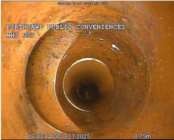
MH3US3X_3f4a6527-1d2c-4c5c-a04e-ee7332cf6774_20251030_155956_697.jpg, 00:00:07, 0.75 m Junction at 9 o'clock, 100mm dia
