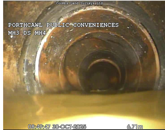
MH3X_f3c677d4-5b37-4da2-ba64-9a5289535fb3_20251030_163614_646.jpg, 00:02:19, 6.71 m Pipe material changes to polyvinyl chloride at this point
