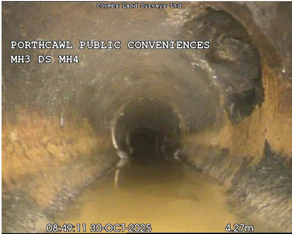
MH3X_60c0f3d8-877a-499b-9ba9-6412a4587609_20251030_163305_780.jpg, 00:01:43, 4.27 m Junction at 2 o'clock, 100mm dia
