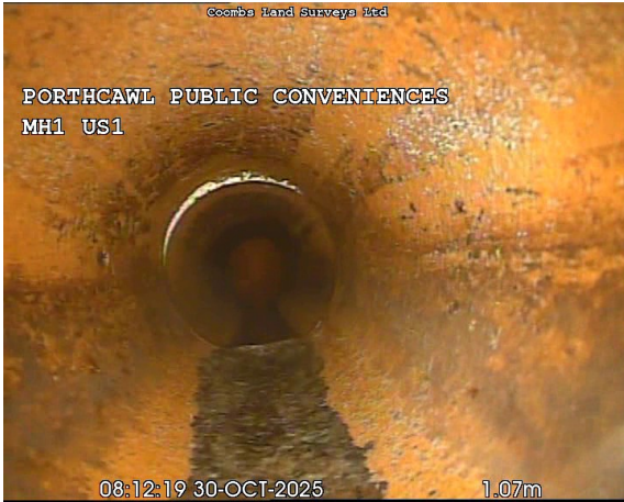
MH1US1X_55b3ed35-e792-439d-9ae8-b72801b28589_20251030_134838_261.jpg, 00:00:15, 1.07 m General photograph taken at this point
