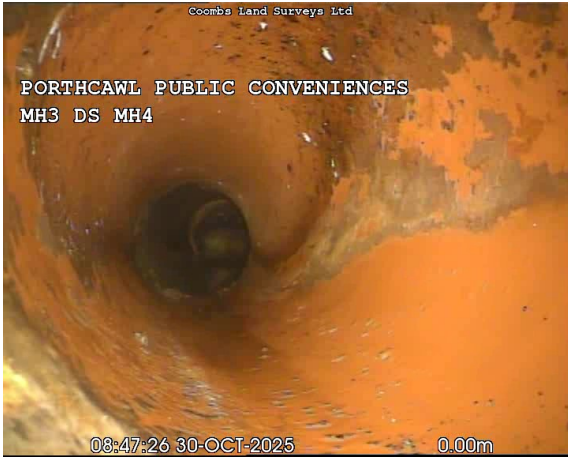
MH3X_418307b6-13d7-4593-ada3-9e94e3167a6f_20251030_161407_742.jpg, 00:00:00, 0.00 m Pipe material changes to polyvinyl chloride at this point
