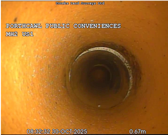
MH2US1X_490efec0-cf34-4e2c-b150-a3c6d1312257_20251030_143816_970.jpg, 00:00:17, 0.67 m General photograph taken at this point
