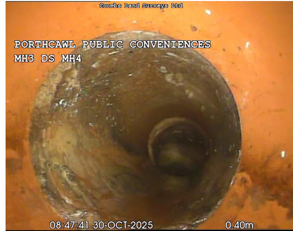
MH3X_b5803963-3c9b-4e64-8e15-a707f72d7986_20251030_161505_988.jpg, 00:00:14, 0.40 m Pipe material changes to vitrified clay at this point
