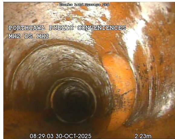
MH2X_e4d69121-2443-47b6-abbd-9630be055c17_20251030_152957_817.jpg, 00:01:14, 2.23 m Junction at 3 o'clock, 100mm dia
