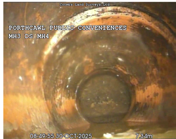
MH3X_bf86b677-1983-4596-8939-4c359911e1e4_20251030_163714_623.jpg, 00:02:28, 7.34 m Pipe material changes to vitrified clay at this point
