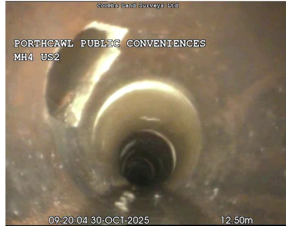
MH4US2X_2ae1a038-8453-4358-a1cf-b82174d65e0b_20251031_091821_216.jpg, 00:01:15, 12.50 m Connection other than junction at 10 o'clock, 100mm dia
