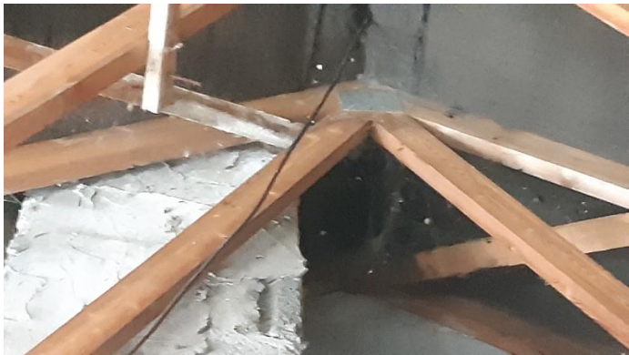
Fig. 11 Southwest gable end, northwest pitch
