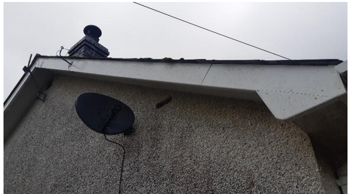
Fig. 4 Tiles tight over southwest gable, southeast pitch
