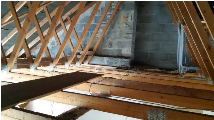
Fig. 9 Sealed wall top, southwest gable end
