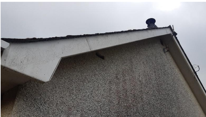
Fig. 5 Tiles tight over southwest gable, northwest pitch
