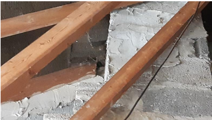
Fig. 10 Showing sealed wall top under southeast pitch
