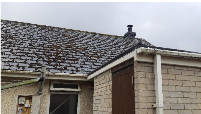
Fig. 7 Northwest aspect, north end and store roof
