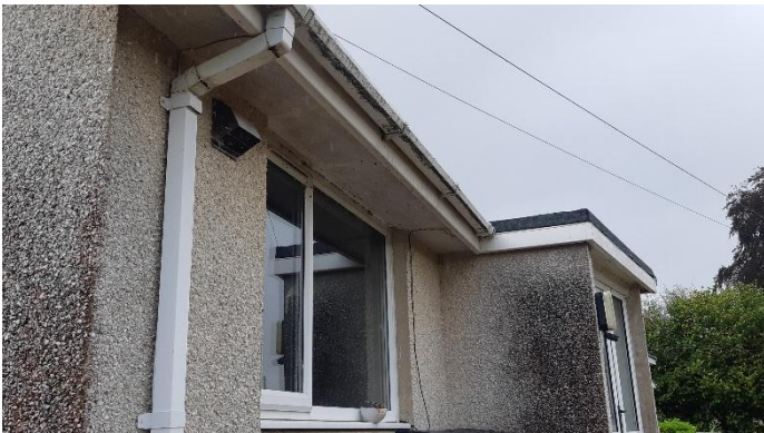
Fig. 3 Sealed soffits and fascias, southeast aspect
